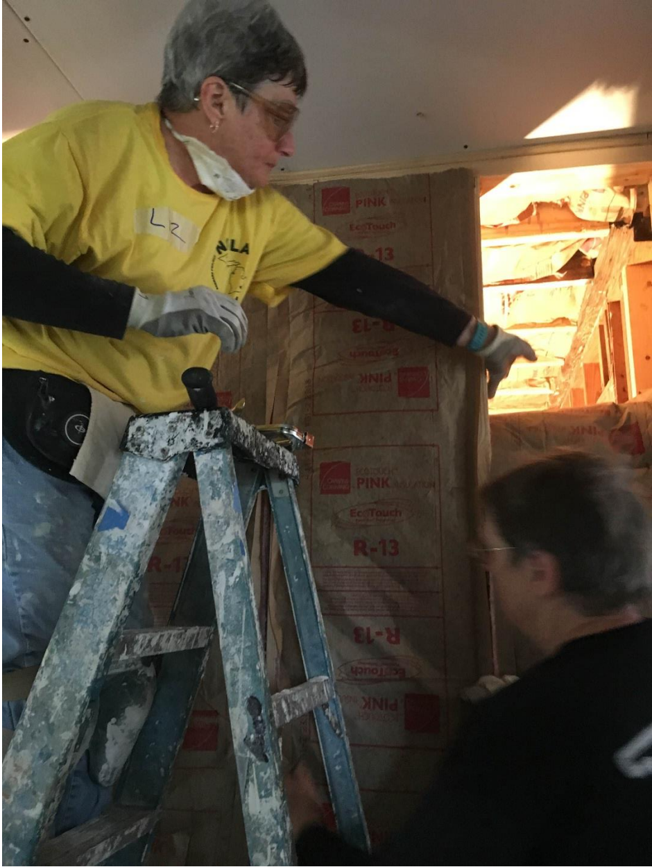
Installing insulation
