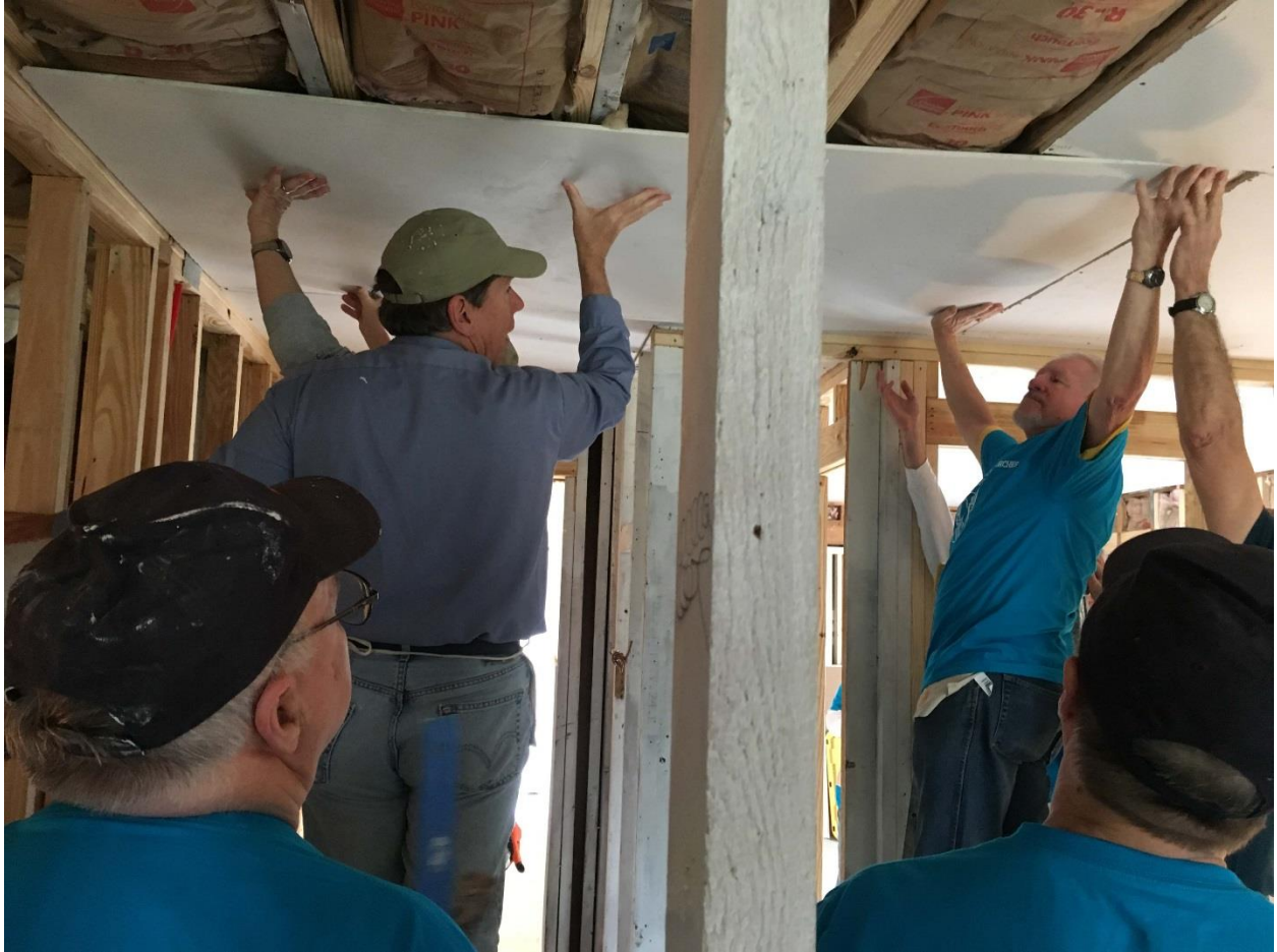
Installing ceiling panels
