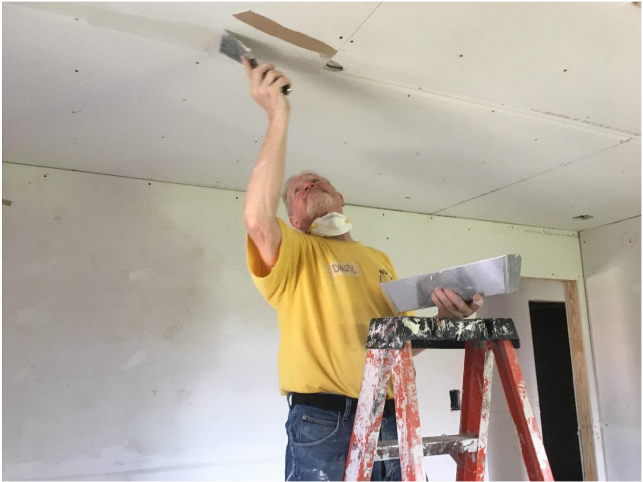
“Mudding” to cover joints and imperfections in newly-installed drywall
